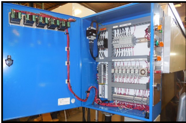
ULTRA VS-6 LE—Electrical Panel with sophisticated temperature display & Indicator light system
